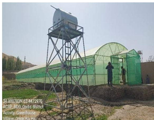
Greenhouse Constructed, Qadis and Bala Murghab districts, Badghis Province are operational
