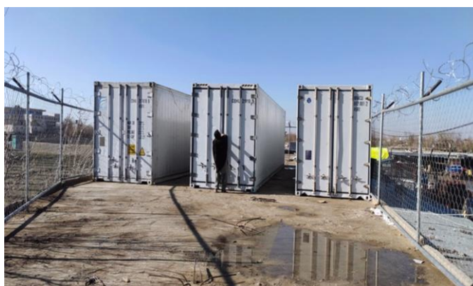
Installation of three reefer units covered with fence at Al-Sadat Sabzi Market, Greshk District, Helmand province, 29-Dec 2025.
